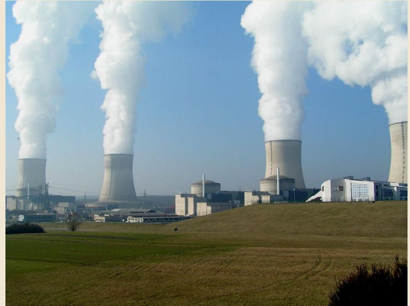
Cattenom Site (4 nuclear reactors)
